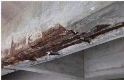
The detection of the hot spots where active corrosion begins involves the measuring of the localized negative values of the half-cell potential (i.e. corrosion potential). When using a rod electrode the user has to define a grid fine enough not to
